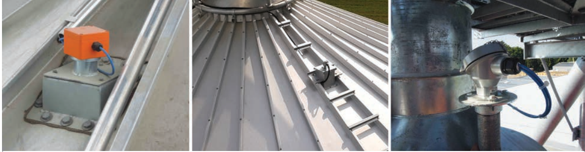
Picture 7, 8 and 9: T-monitoring solution in metal silos Resim 7, 8 ve 9: Metal silolarda T-izleme çözümü
